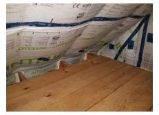
3. *Tip from the Field* – When insulating the slopes of a cape-style home, be sure to extend the insulation and air barrier below the level of the floor and to the top of the first floor wall, as shown in the adjacent picture. This often requires removing a portion of the flooring to access the space between floors.
